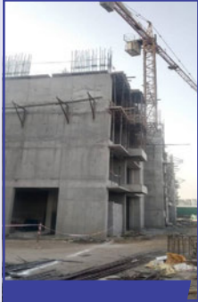
(Mar - 21) 4 th Slab
