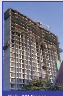
(Feb- 22) Super Structure Completed
