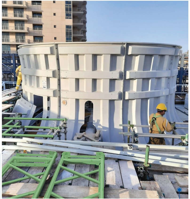
Cooling towers being installed by Blue Star at 'Gewan District Cooling Plant Project,' the Pearl-Doha, Qatar
