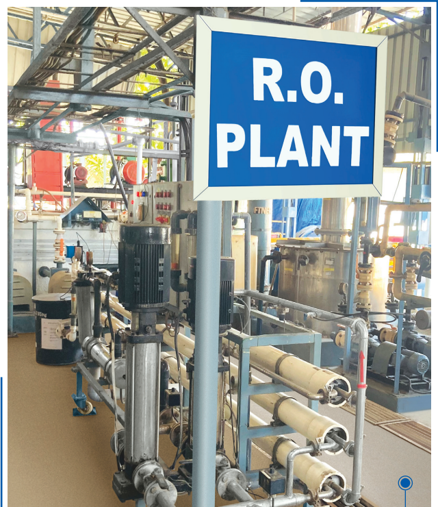
Reverse Osmosis (RO) Water Treatment Plant at Blue Star's Dadra manufacturing facility
