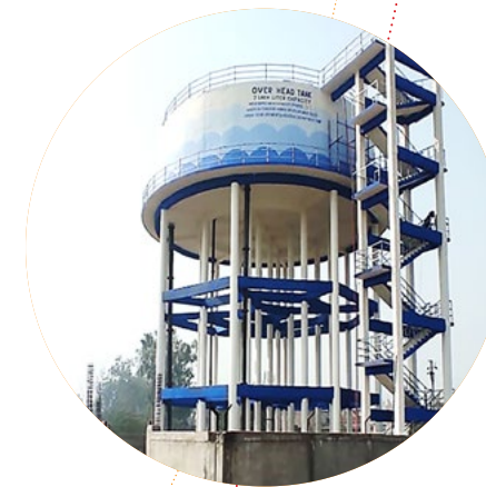
Bhind Water Supply
