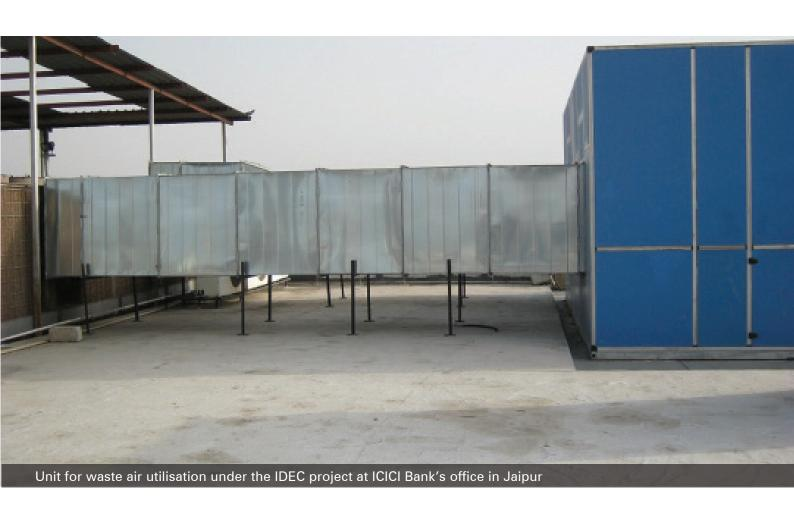
Additionally, the waste air from the IDEC is being used to reduce the ambient temperature of the chiller. A duct has been created from the IDEC to the chiller. Cool air at 16 degrees from the blowers is supplied to the chiller through the ducts. This innovative use has led to 34,800 cubic feet per minute (CFM) per hour of cool air being used to reduce the ambient temperature of the chiller. It has contributed to up to 50% saving on power consumption of the chiller.
